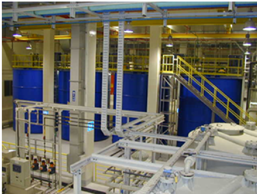
Figure 10: Wastewater Treatment Plant
