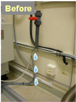
Potential oil leak causing hazards
